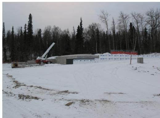
is drilled and capped, and underground utilities are complete for the major utilities. The slab in the mezzanine was poured in December 2009 which will allow the boiler to be installed in January 2010. This will keep construction going through the winter putting this project ahead of schedule. Pre-engineered structural panels are expected to start arriving in April 2010, at which time the structure will be erected. The project is on schedule for an October 2010 completion.
