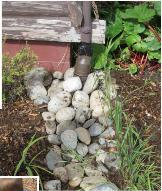
We buried a gutter extension in a rock trench to bring stormwater input away from the foundation and into the rain garden.
