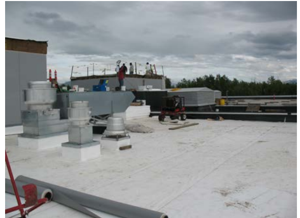
ABOVE: Roof work on another district school
